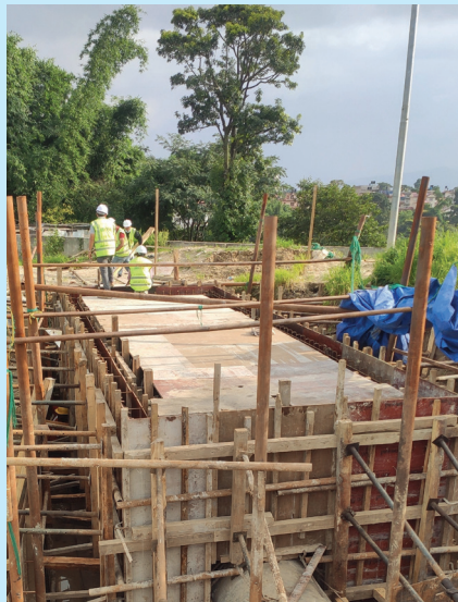
■ Construction of RMU Chamber at New Bansbari, Kathmandu is in progress
